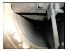
**9.4** The fresh air intake is clogged with debris. *I recommend cleaning off and checking on a monthly basis. Repair as desired.*
