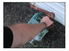
**7.6** The sump pump worked fine. I recommend to keep clean from debris and test monthly for function.
